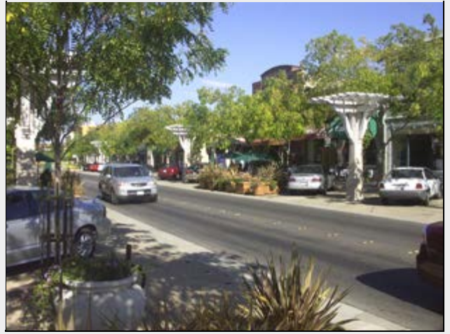
Sustainable downtown revitalization: 1st St., Livermore, CA (Credit: Greg Tung, Freedman, Tung & Bottomley).
